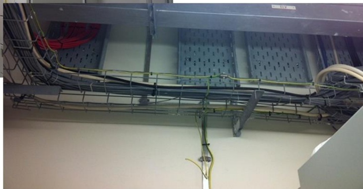
Unused cable trays in the basement North Riser.
