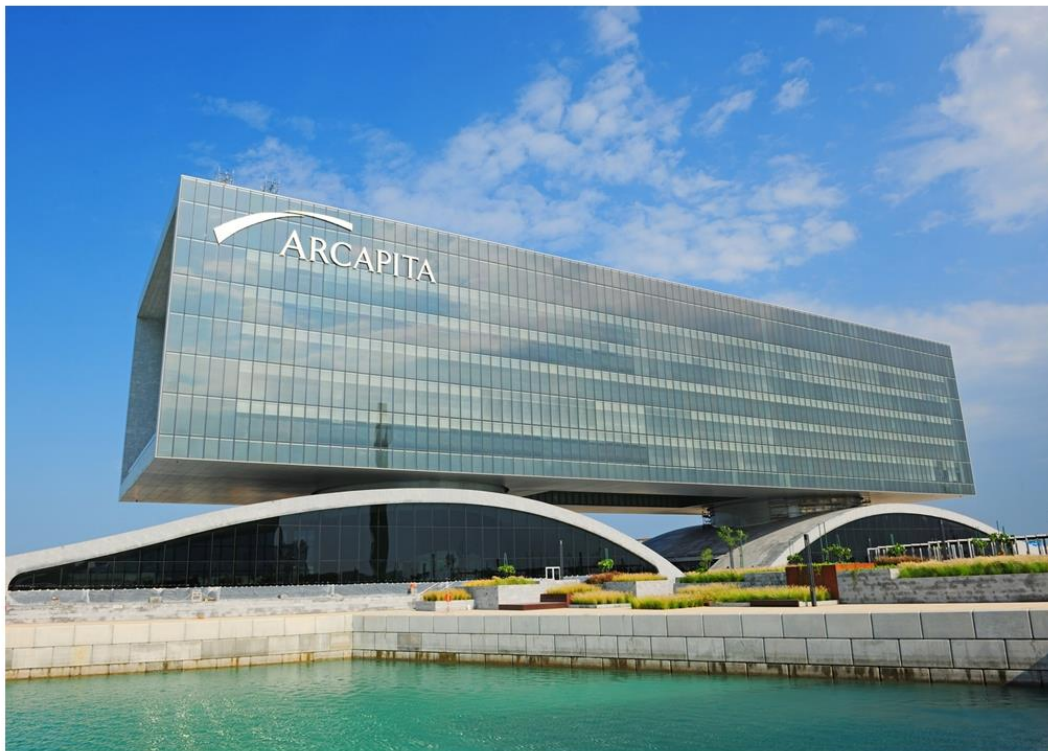
Arcapita Bank Building, Bahrain, equipped with a fully integrated enterprise and building management network infrastructure
