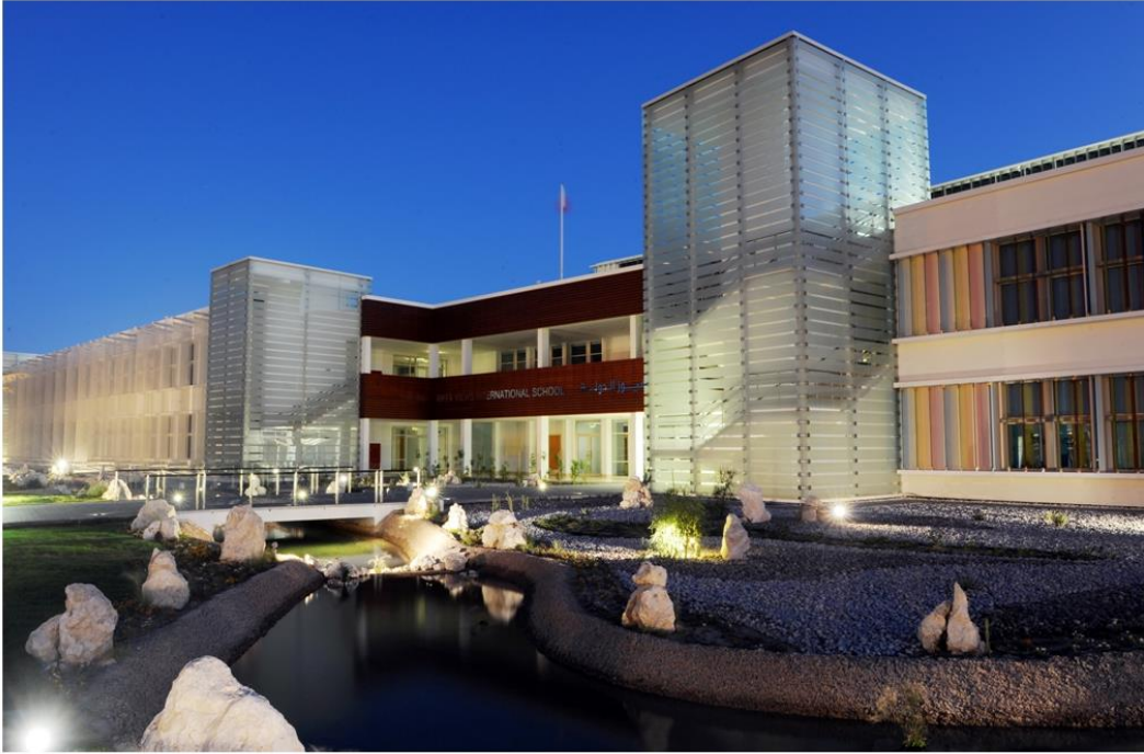
Riffa Views International School, Bahrain, featuring a cloud network infrastructure and wireless classrooms
